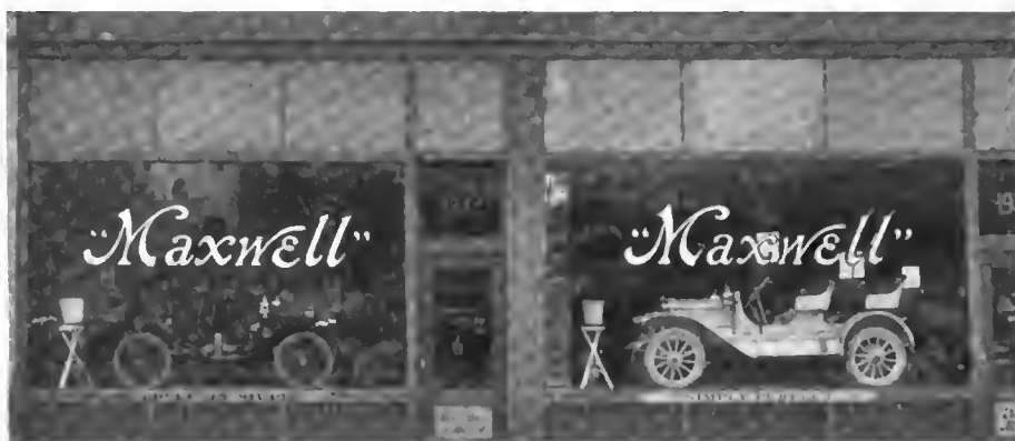
New Quarters of Maxwell-Briscoe Motor Company at 1930 Broadway, New York City.
